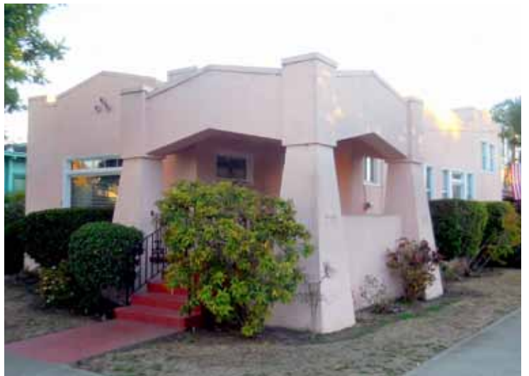
2700 San Jose Avenue (1919) , George H. Noble, owner and builder. Noble's bungalows of the late teens often included bold parapets as signature elements. This example is definitely one of a kind.
