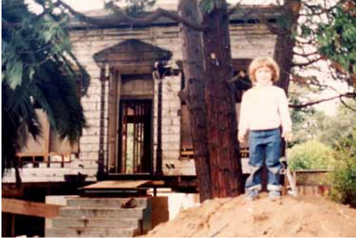
The author's daughter Rachel, age five, at the time of the home's restoration. The dark paint shadows on the front of the house were used to recreate the missing porch and its decorative elements.
