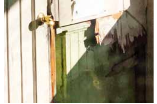
Next to the front door and below the map on the wall, notice that the plaster has been pulled off to show the original paneled woodwork that formed the front low wall of the station.
