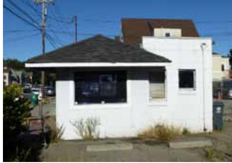
Current forlorn state of affairs for the Webster Street waiting station, January 2017. Note the window openings on both west and east sides confirm the existence of the underlying architectural structure for the original 32 light windows that at one time enclosed the station. The concrete blocks that form the back portion were added later to enlarge the structure and at that point most of the back wall of the station was removed.
