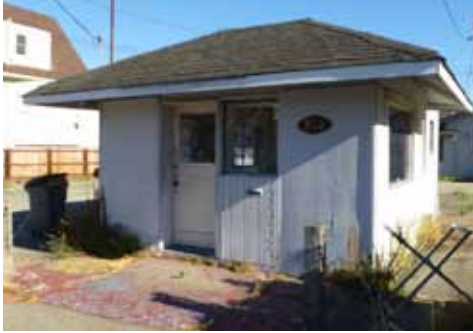
Current forlorn state of affairs for the Webster Street waiting station, January 2017. Note the window openings on both west and east sides confirm the existence of the underlying architectural structure for the original 32 light windows that at one time enclosed the station. The concrete blocks that form the back portion were added later to enlarge the structure and at that point most of the back wall of the station was removed.
