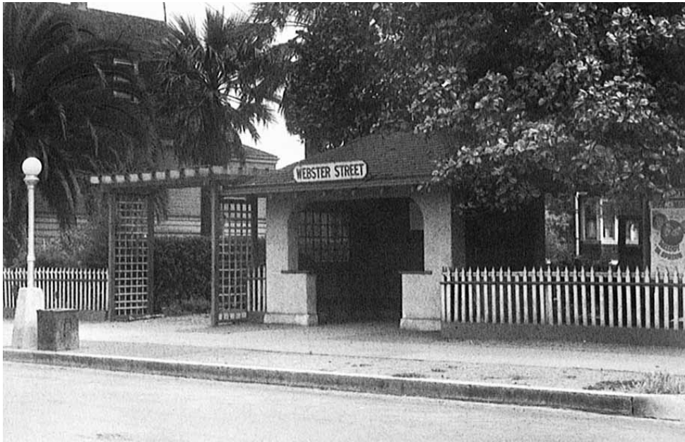
The Mission Revival station shelter in its original setting. The billboard seen on the right edge of the photo for the Neptune Palace Theatre, where "Good Dame" and "Melody in Spring" were running at the time, dates this picture to 1934. Image: "Alameda by Rail", by Grant Ute and Bruce Singer.
