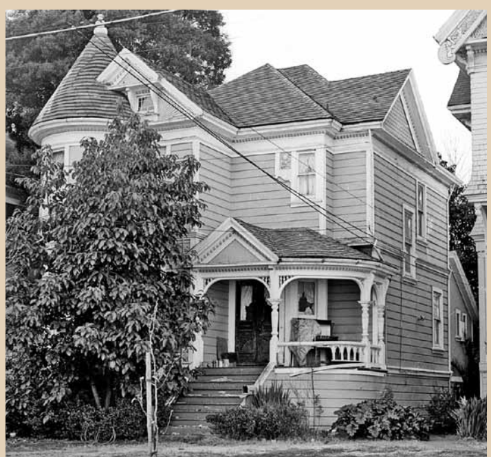
Above: This photograph from the 1979 Survey shows the how grand the home is in size, but it has started to show some neglect. The porch spindles and trim have fallen away, the wood stairs are worn, and the stair railing is missing.
