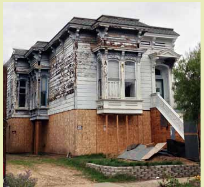
Above: 1315 Mound Street has lost most of its paint at this point. Below the waterline its redwood siding has been removed along with the lower windows, and brackets under the bays. Below: After restoration and a fresh coat of paint. The home was renovated inside and out. Image: Phoebe Yu.
