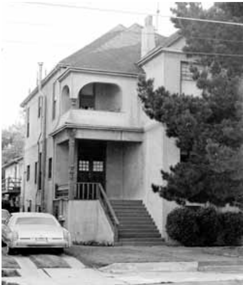
Left: 1833 Clinton Avenue was covered in stucco in an attempt to modernize it in the 1960s.
