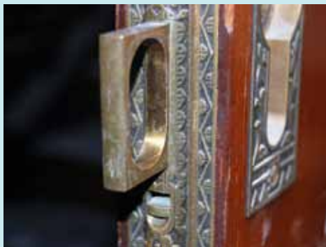
(b) Raising the thumb-slide releases a handle
