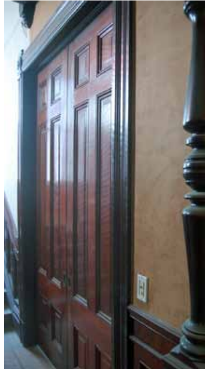
Popular in Victorian-era homes, pocket doors enlarge or enclose living space by rolling into a compartment between walls. They usually travel on rollers suspended on an overhead track or a track on the floor.
