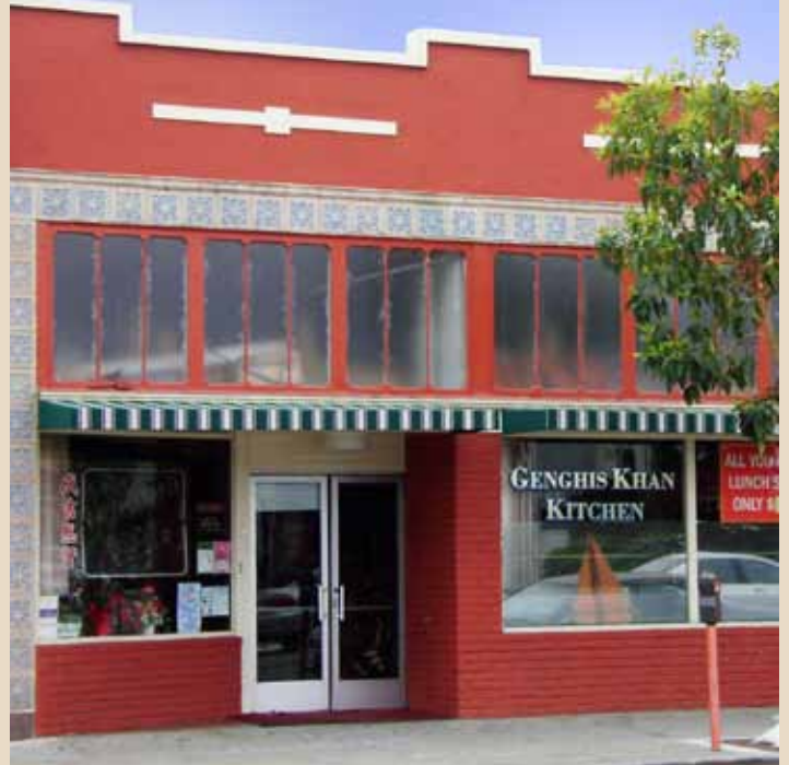
Updates included refreshing the color of the walls, replacing the trim, power-washing the walls and transom windows, and replacing the large awnings, making them smaller as not to hide the upper windows.
