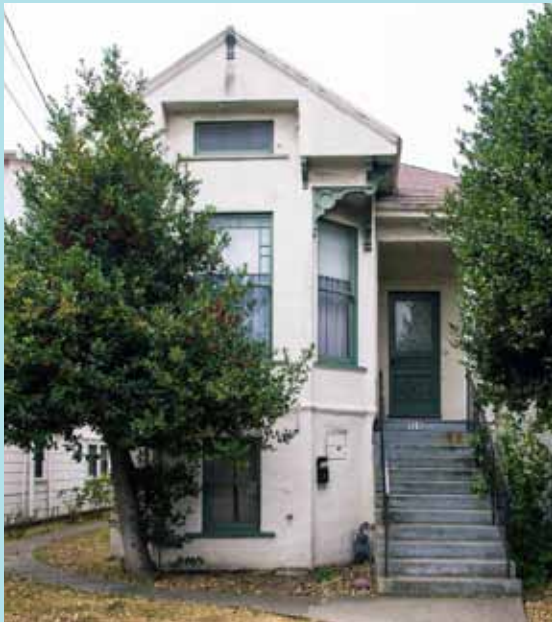
Right: The structure's original beauty is revealed again. Elements that were removed from the house were used in other locations on the property—foundation bricks are found in the front walkway and an ornate gate (above) was constructed from the original porch railings.
