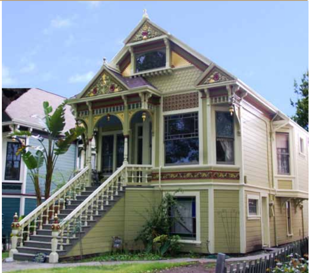
The restoration work at 1530 Mozart Street was coordinated by owner Tommie Veirs acting as her own general contractor. This included restoring the cresting on the roof. This original cresting was discovered in the basement, apparently removed in an earlier roofing job and never reinstalled.
