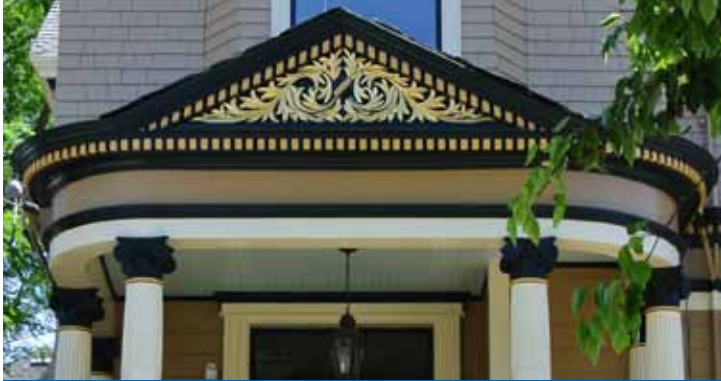
Original elements include the gold leaf relief above the front porch and bay window, the stucco on the front façade, the egg and dart molding around the turret, and the small attic windows and surrounds.
