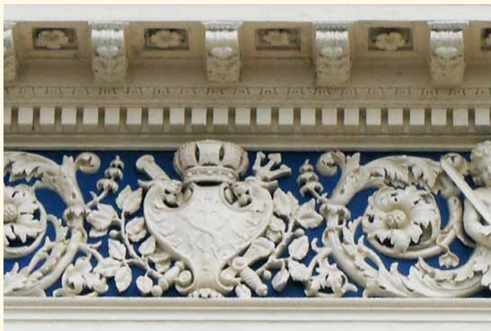
These terra cotta panels formed a frieze on all four sides of the Oxford & Cambridge Club, an exclusive establishment we were allowed to tour... as long as we were "smartly dressed." (Photo Judith Lynch)
