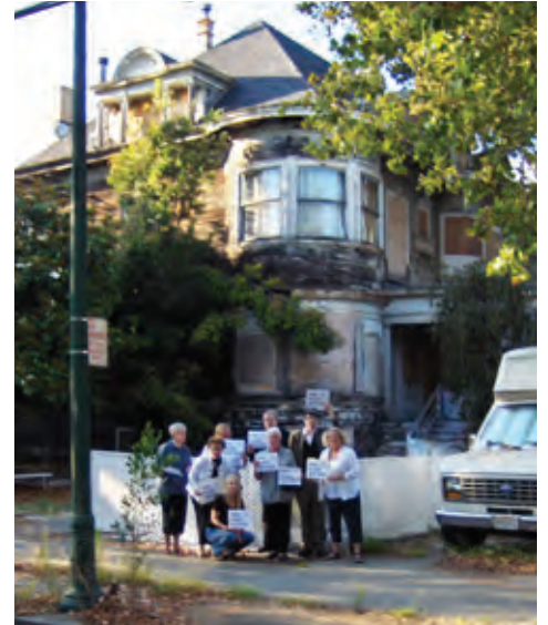
The AAPS Board at 1617 Central Avenue holding "This Place Matters" signage. The 1897 Colonial Revival home has been declared substandard and ordered vacated by the city. (Photo Thom Mantooth)
