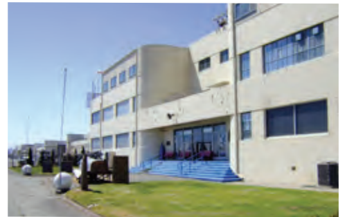
The NAS Air Passenger Terminal was where "VR" Squadrons operated from. The squadrons transported passengers and freight between Naval Air Stations all over the world. It is now home to the Alameda Naval Air Museum. (Photo Valerie Turpen)
