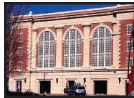
Staunton, VA Parking Garage
