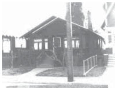
*Approved by the Planning Department in 1993. Second story added, front porch partly enclosed and entire building covered with vinyl siding. Original surfaces were wood shingles. Horizontal aluminum slider windows added which are inconsistent with the original Craftsman style*
