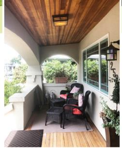
Natural Douglas Fir tongue and groove was used on the floor and ceiling of the new porch.
