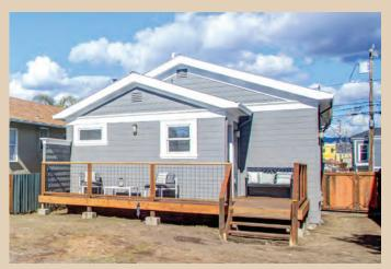
In order to enlarge the attic, the hip roof at the rear of the house was changed to a gable roof.
