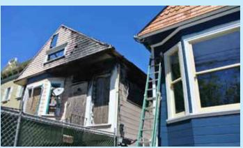
Right: Melted siding revealed original wood shingles underneath.
