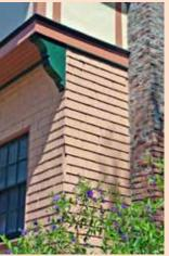
The Home of Truth features Arts & Crafts details such as half-timbering, shingles, wood brackets, and clinker bricks.
